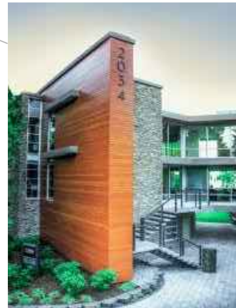
WOOD SIDING- PORCH COLUMN OR FULL WALL
